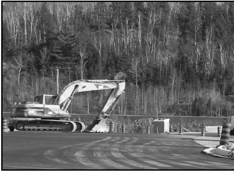
Work on the Levack/ Onaping Water Line
