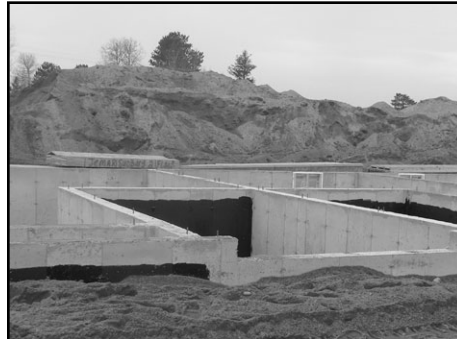
New foundations in Levack, Kastletree Homes starts construction
